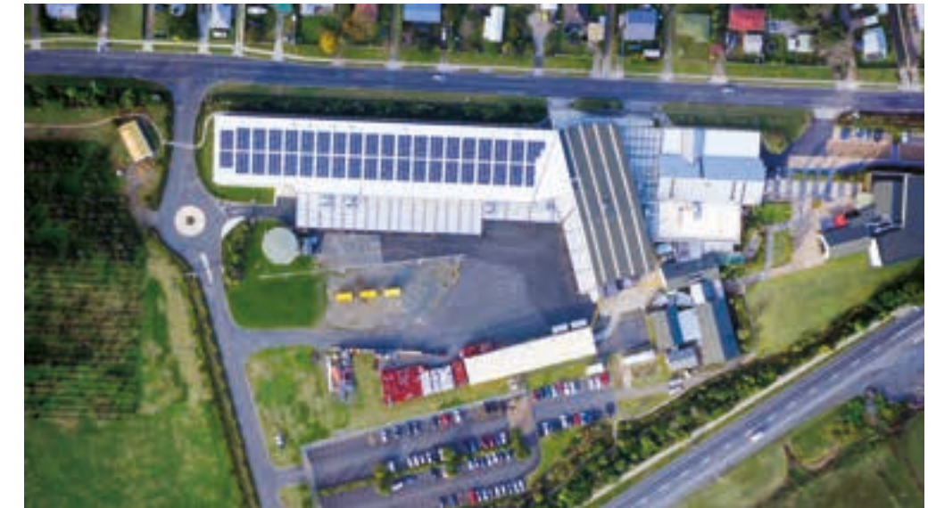
Solar panels on our 23 Wilson Road South Paengaroa hive.
